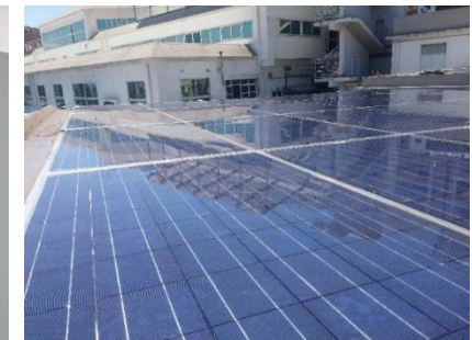
PV policristalline roof top plant P=3kW
