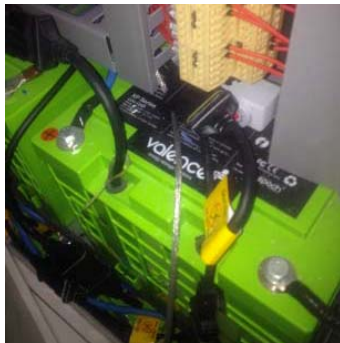
LiFeMgPO 4 Batteries Energy =5 kWh
