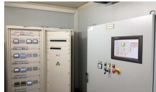
Control panel and bidirectional AC/DC converter
