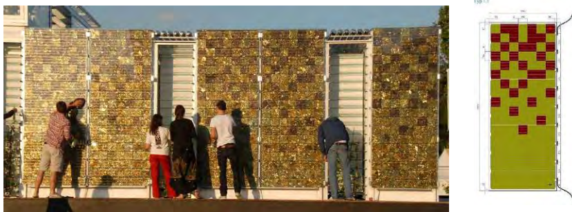
Fig 3.6: home + pavilion for Solar Decathlon, photo of façade and technical drawing of a façade module, ©Prof. Dr. Jan Cremers
