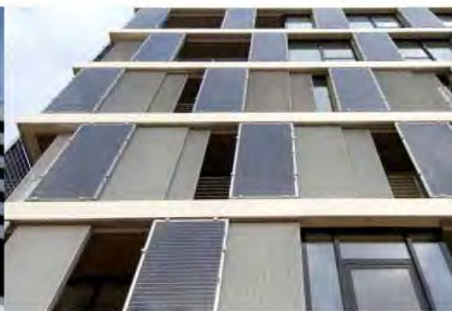
Colt Ellisse PV sliding shades at Company HQ, Bitterfeld-Wolfen, Germany, © Colt International Licensing Ltd., 2011
