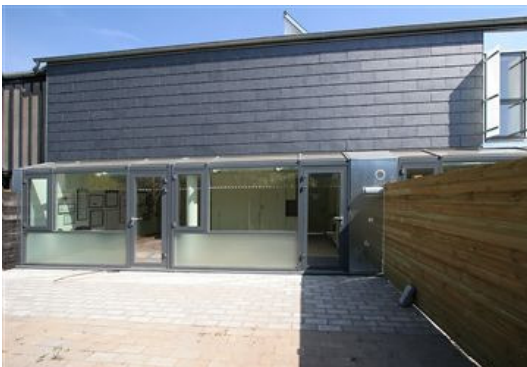
Bay windows – seen from the garden
