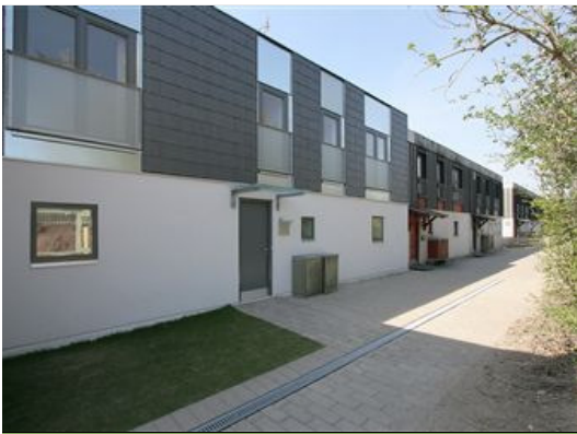
House 15C – after the renovation
