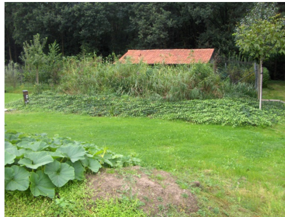
Reed field for wastewater treatment
