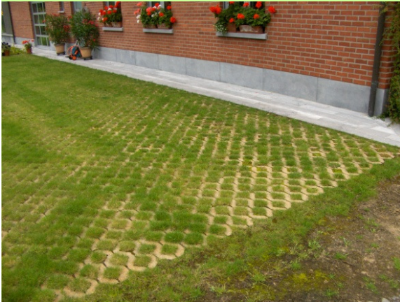
Special tiles enable for rainwater absorption
