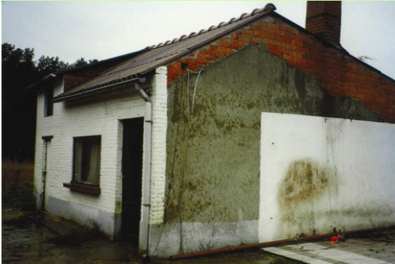
The garage before the renovation
