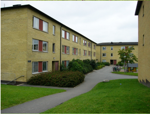
Brogården before renovation
