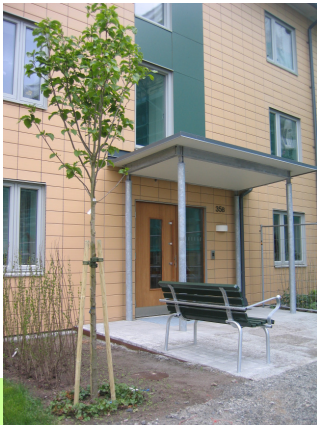
Entrance after renovation
