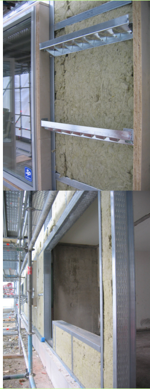
Outer wall with its layers of insulation
