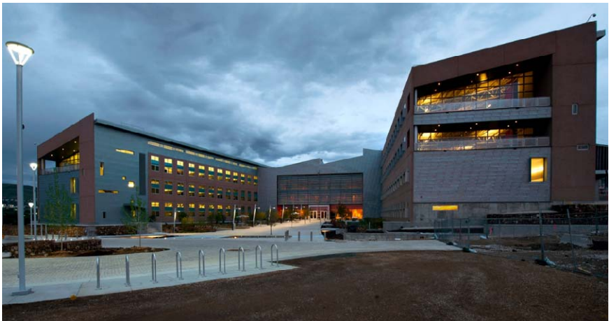
NREL Research Support Facility, Colorado
