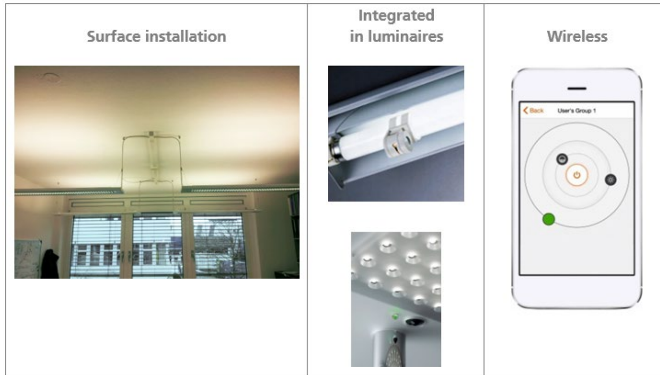
Figure 19 | Compilation of the possibilities for upgrading lighting management. [© Fraunhofer IBP, Nimbus, Osram]
