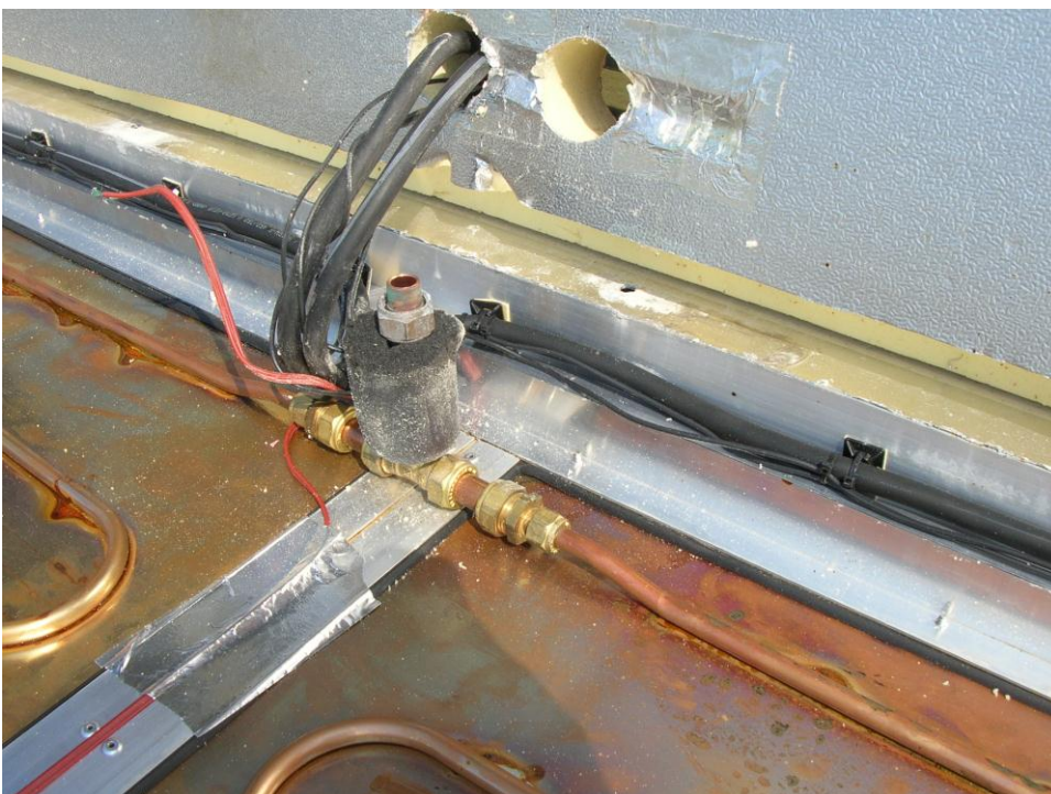
Figure 2. Compression T-joint and cabling details
