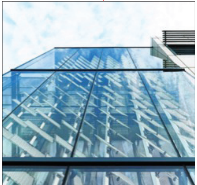
Upward view of the demonstration facade of the lumiduct BIPV system (Source: Wellsun).
