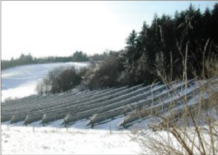
▲ Figure 3. First solar district heating system in Denmark: SALTUM 1988, 0.7 MW, 1,000 m 2 . The system remains in operation in 2011.
