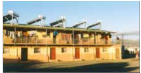
▲ Figure 2. Mass rollout, stand alone solar thermal water heaters.
